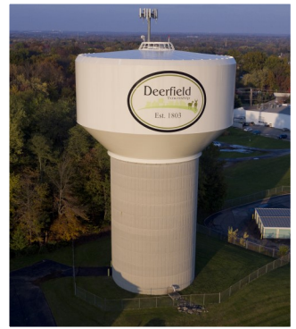
20 Mile Elevated Water Tower
