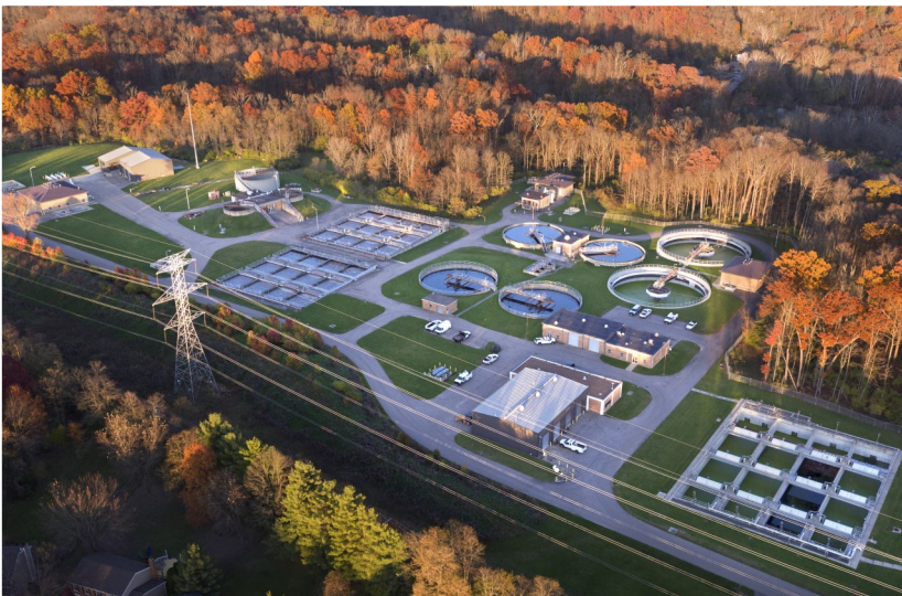
Lower Little Miami Wastewater Treatment Plant
