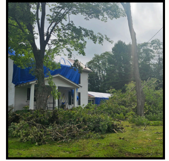
July 30th Tornado Damage Assessment
