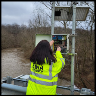
Maintenance on EMA River Gauges
